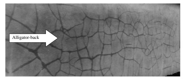
Several factors may contribute to this loss. When fresh plaster is direct-applied to a solid substrate (concrete, block, stone, brick) the substrate should be dampened to prevent the type of cracks shown above.
