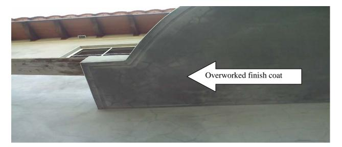
It may be unwise to try to seal all of these cracks and it is generally considered inadvisable where cosmetics are the only reason for doing so. These minor cracks are usually more pronounced after a rain or on a foggy morning as the wall begins to dry out. Often, the repair of this type of crack is more visible than the crack itself. The owner should decide which direction to go.
