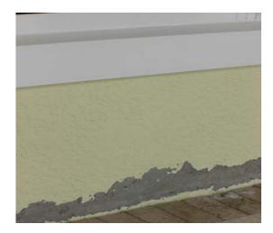
Severe alkaline burn results in saponification. The mottled or blotchy appearance of coatings is only the first symptom of high pH. High pH combined with water may also cause saponification or, in layman's terms, the breakdown of the coating from behind
